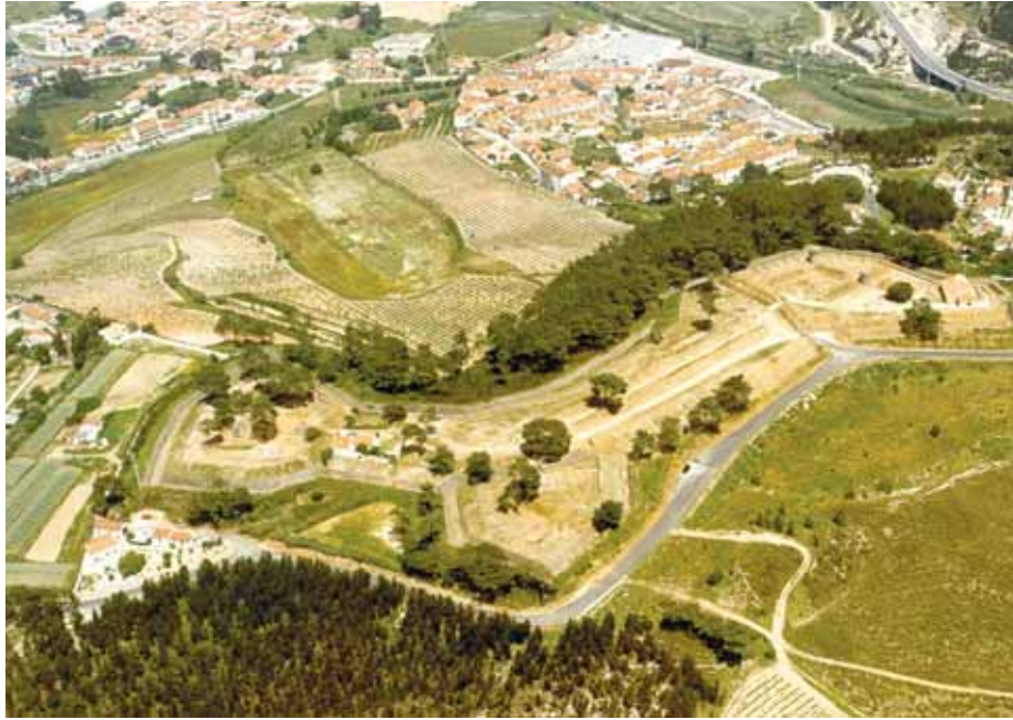
Figure 16 – An aerial view of Forts 20, 21 and 22 comprising the main redoubt at Torres Vedras (São Vicente) which was situated to the north of the town and the River Sizandro. This is the only fully restored redoubt on the Lines. The work was done by the Portuguese Engineers under Colonel Francisco Baptista in the 1960s as recorded in an article in the Royal Engineers Journal (Vol 25, No 4, December 1961). (Courtesy the Portuguese Ministry of Defence)
