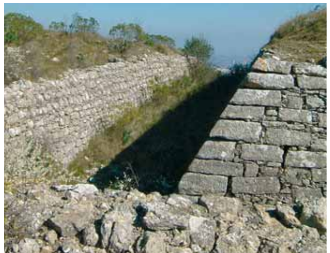
Figure 10 – An example of fine stonework in Fort 40 near Alverca.
